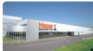
1983 Yamazaki Mazak Manufacturing Corporation, Minokamo Plant
